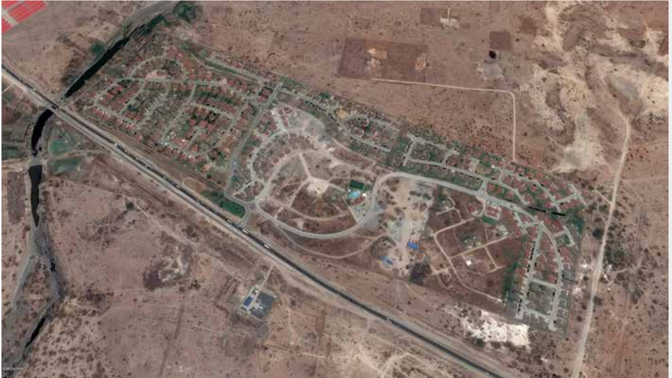
FIGURE 4.11 An isolated housing development south of Nairobi along Mombasa Highway
